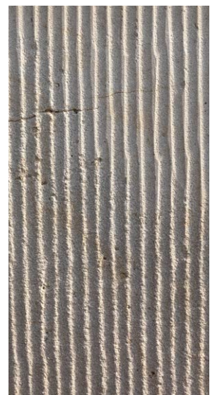
Detail of a wall, Vindebrogade
