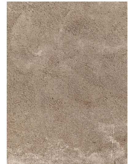
Detail of a wall, Christiansborg Slotskirke
