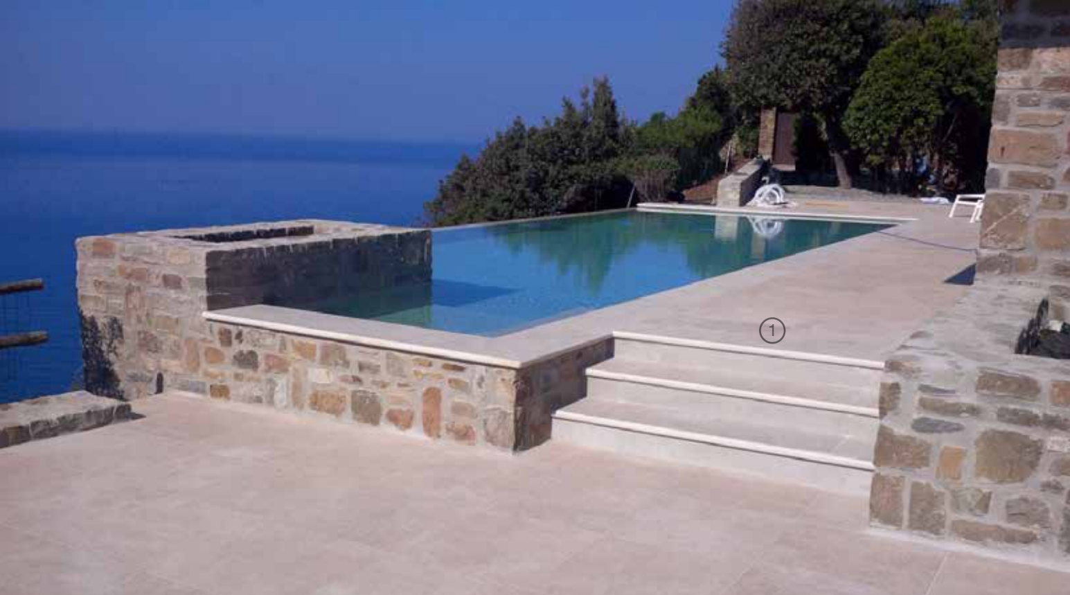
STAIRS AND FLOOR GREIGE 2.0
